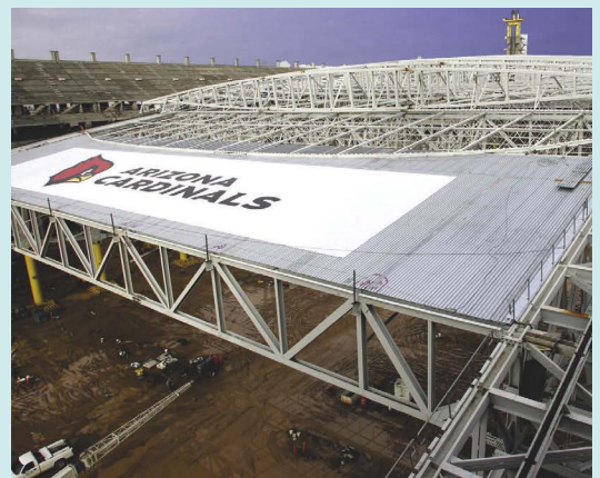
Chicago Metal Rolled Products curved 402 tons of 12" square tubing for the retractable roof of University of Phoenix Stadium in Glendale, Arizona.
